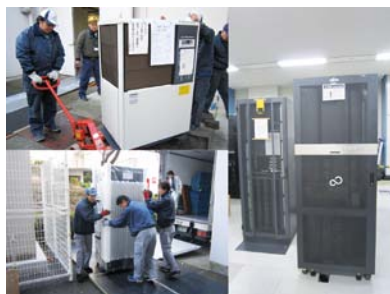
Fig. 1 : SCLS computer system installation field site of
