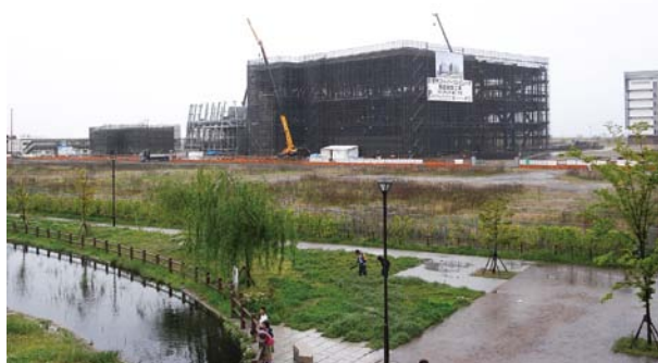
Building of Advanced Institute for Computational Science under construction (April, 2009)
